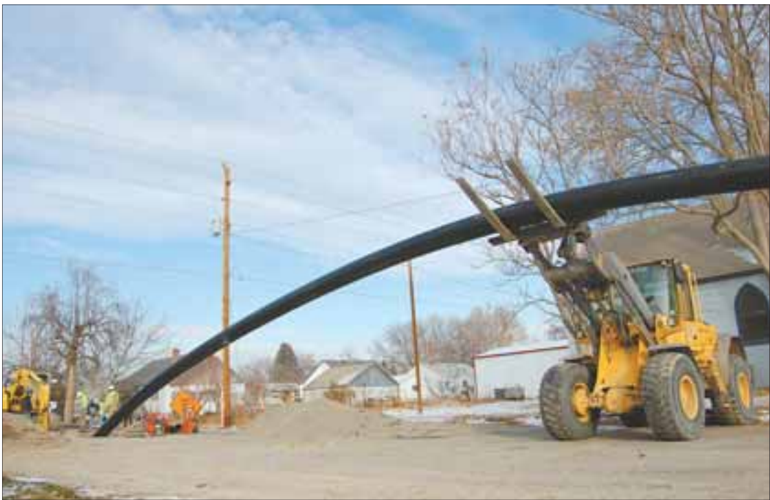
A long stretch of pipe spans North 1 st Street East near its intersection with East Owyhee Avenue as crews continue to rehabilitate sewer mains throughout Homedale.
