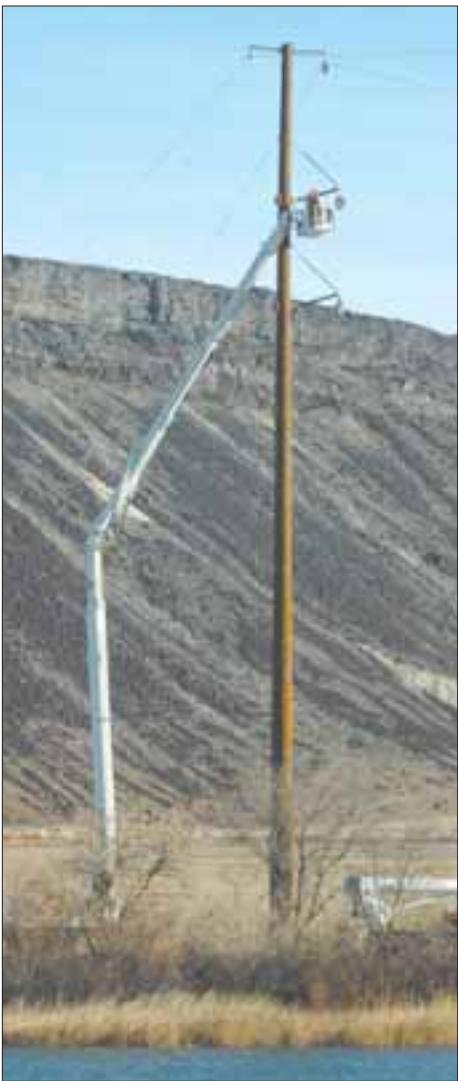
Idaho Power workers secure part of the Bowmont-to-Hemingway 230-kilovolt powerline to a pole standing on the Canyon County side of the Snake River.
